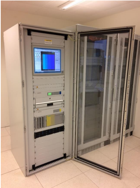
Fully integrated rack solution with DTS, DAS and SmartVision™ in the control room
