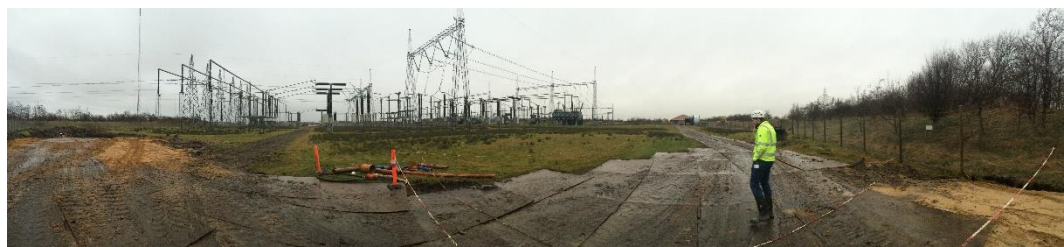
Underground cable route inspection
