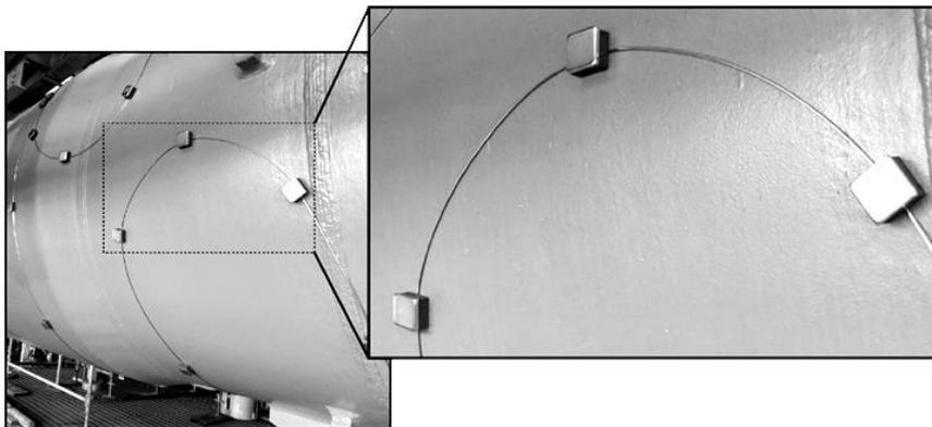
Fig. 1. Stainless-steel sensor cable mounted on a reactor skin using high-temperature magnetic fixtures.
