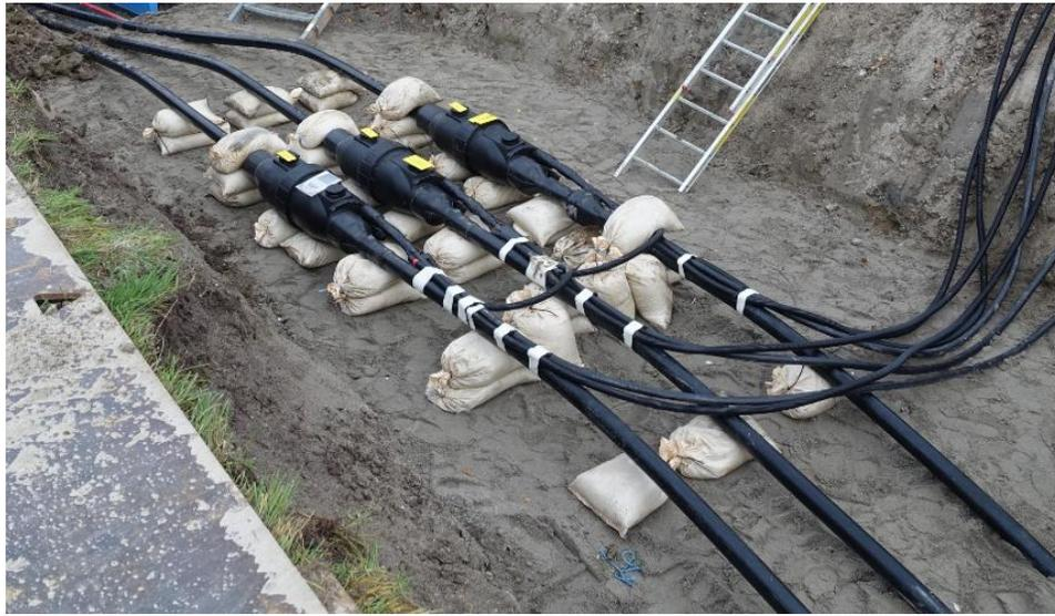
Figure 1: Example of cable joints in a joint pit for three separate phases
